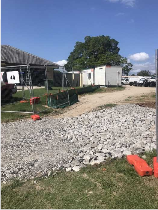
Image 1: Construction site and heavy earthmoving. See truck entry point.
